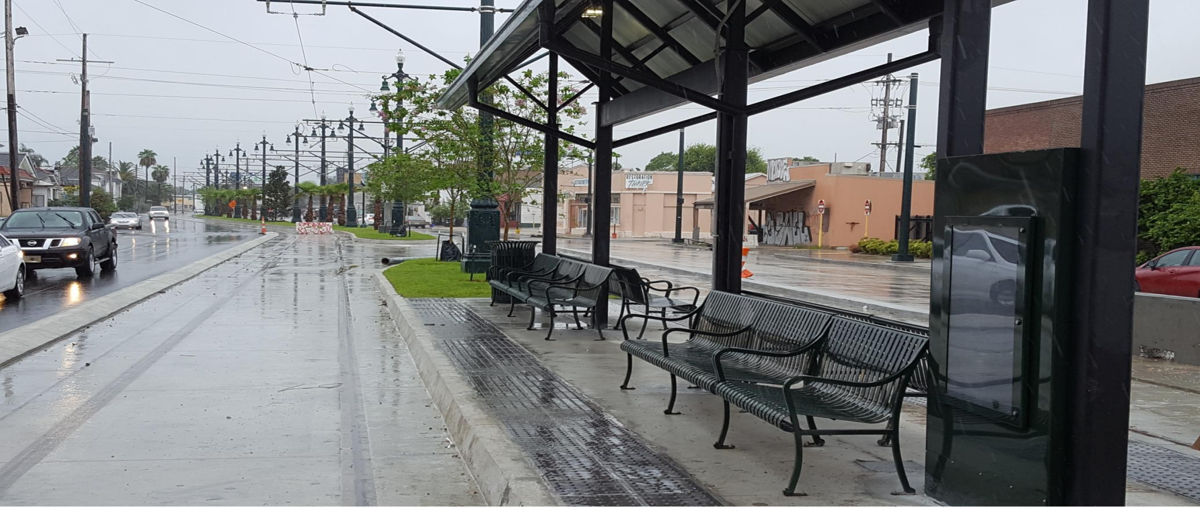
Elysian Fields Streetcar Stop looking down towards Canal Street
