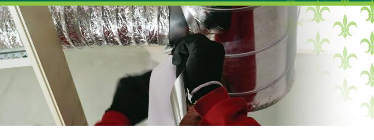
The Small Commercial Duct Efficiency program is designed to overcome market barriers that prevent commercial customers from having HVAC duct systems properly sealed. In ducted HVAC systems, 20 to 30 percent of the air you pay to heat or cool your space is wasted due to leaks. By identifying and sealing leaks with special foil tape and airtight mastic, your trained contractor will save you energy and money and make your system more efficient.
